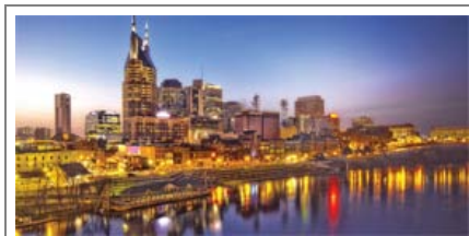
Downtown Nashville's skyline has been transformed by new skyscrapers the past several decades.
